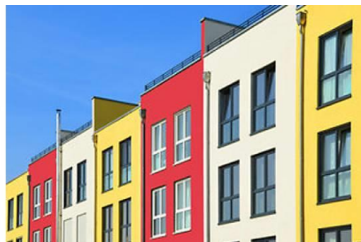
Glass bead RR materials applied to building facades
