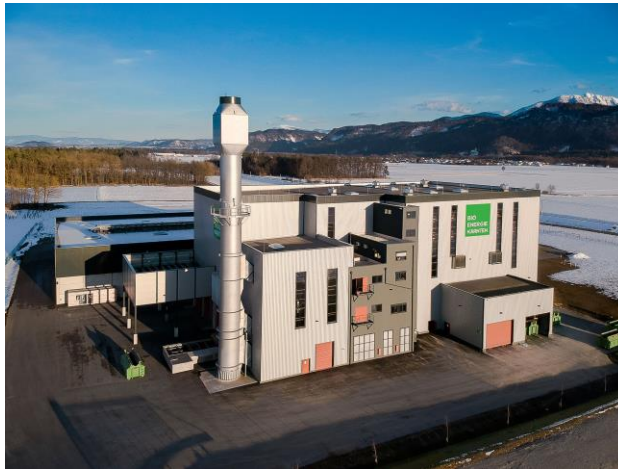
Biomass Power Plant
