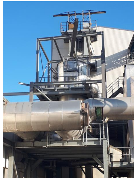
Waste Gas Heat Exchanger
