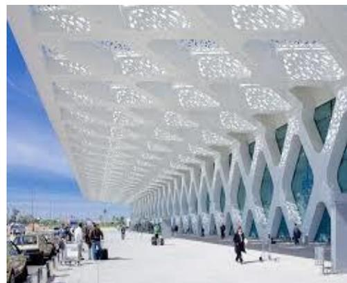
The insulated glass dominating the project incorporates intelligent solar control coatings as Guardian SG HP Bronze 40/27 and Climaguard Premium combined with laminated, tempered and printed glass which contribute to the safety of the building, as well as to guarantee the acoustic insulation.
