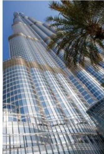
On the Burj Khalifa project, there was the challenge of the temperature difference between the production and installation temperatures of the IGUs. Glass for megatall buildings (i.e. skyscrapers over 600 metres high) often tends to be taken for granted in terms of its technical functions. Yet the high-tech, high strength glazing that covers today's megatall buildings – such as the Burj Khalifa in Dubai – is as important to the building's performance as the steel and concrete inside it.
